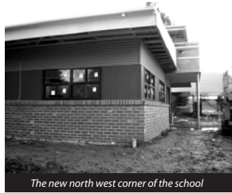
The new north west corner of the school
